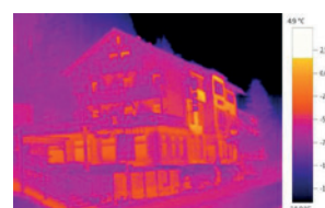
Thermal image with ScaleAssist
